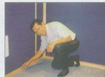
3. Acoustic contractor checking the wall treatment
